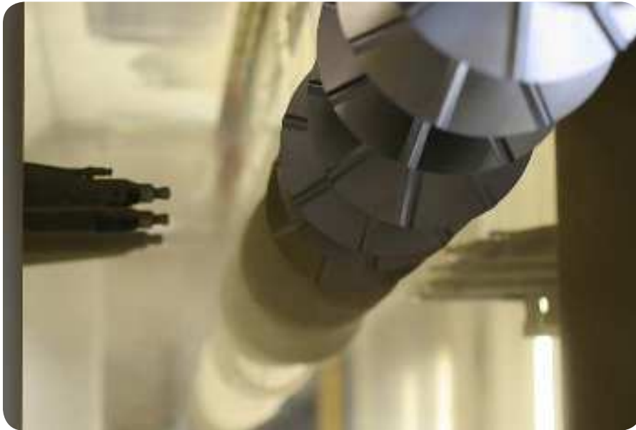
Paint line conveyors are supported by wheels equipped with graphite lubricated bearings.
