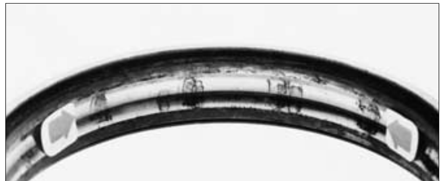
54: Corrosion pits in the raceway at rolling element pitch
