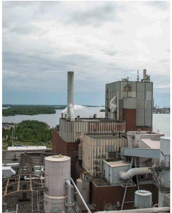
Sunila Mill , Kotka, Finlandia
